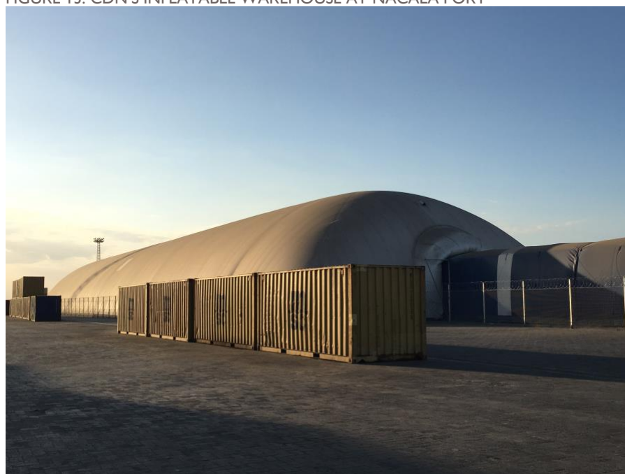
FIGURE 13: CDN'S INFLATABLE WAREHOUSE AT NACALA PORT
